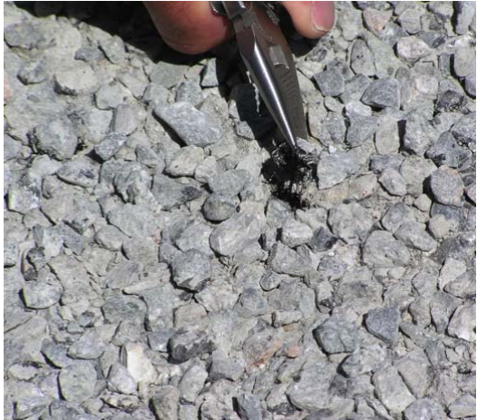
Figure 20. A basic goal is to achieve 50% chip embedment into the binder. This shows an embedment of about 50% which is good.
