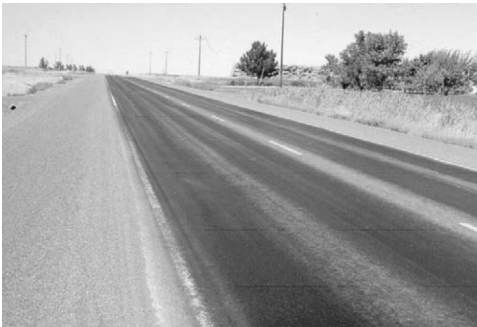
FIGURE A Bleeding or flushing
