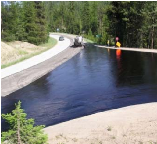
Figure 17. The emulsion color turns to black after it is said to have "broken."
