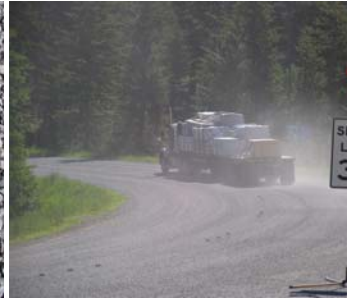
Figure 40. Final BST the next day after brooming. Note reduced speed.
