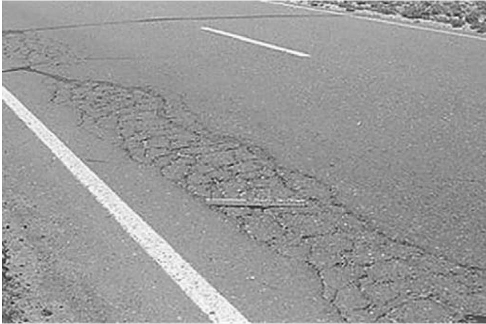
FIGURE 3 Advanced stage of fatigue cracking.
