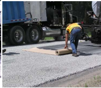
Figure 43. Place the paper at the joint.
