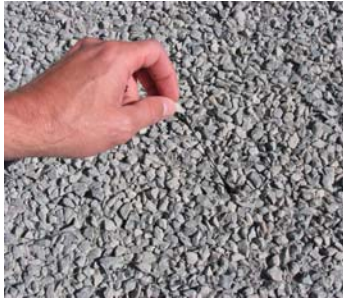
Figure 39. Pulling a rock out showing elasticity of CRS-2P emulsion. Notice long "string".
