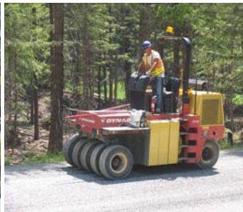
Figure 24. Embedding the aggregate into the asphalt using a pneumatic tire roller.
