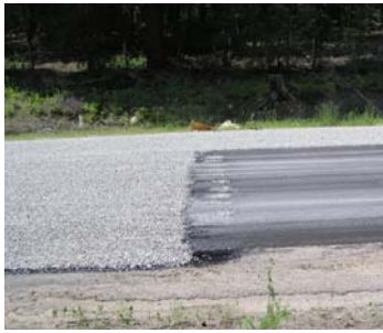
Figure 41. At the end of day, work is stopped and a construction joint is made for continuing the work the next day.
