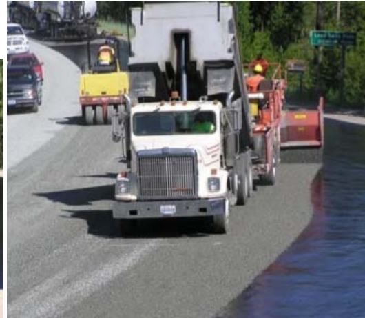
Figure 18. The aggregate should be added to the emulsion before the emulsion breaks. Note that in this photo, the aggregate was added too late, which is poor procedure.
