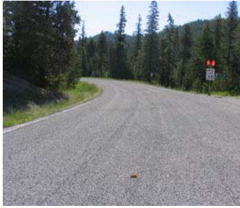
Figure 38. Finished BST before brooming.
