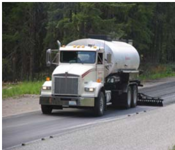
Figure 22. Spray truck applying CRS-2P emulsion at a shot rate of 0.02 gallons/square yard (later increased to 0.08).
