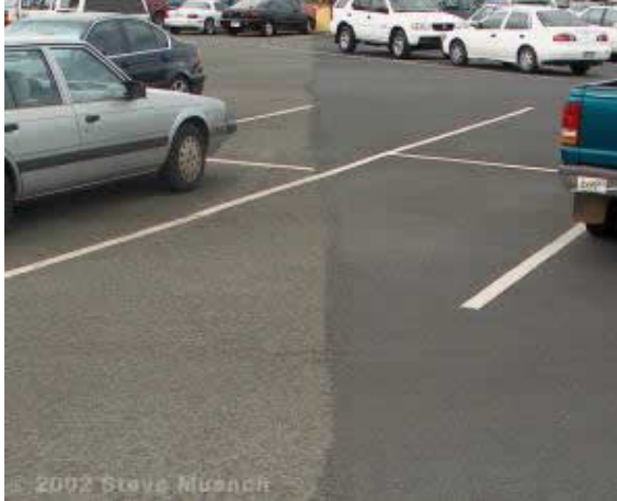
Figure 30: Parking lot showing no treatment on the left side and a fog seal on the right side.
