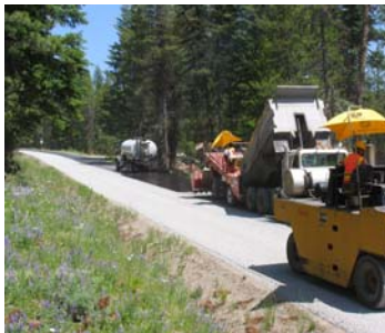
Figure 23. 1/2 inch minus chips being placed - note that the truck is driving backwards as is standard.
