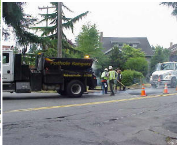
Figure 29: Semi-permanent pothole repair
