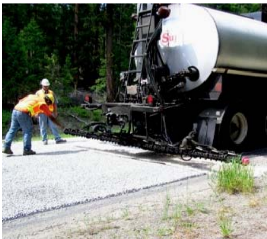
Figure 44. Position the emulsion sprayer to start the shot on the paper.
