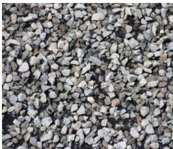
Figure 25. Close up of BST before choke stone application. Not all BSTs use choke stone.
