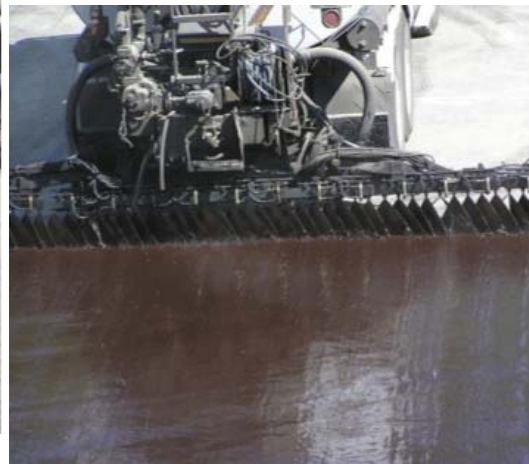
Figure 11. The emulsion spray bar in action. Note the distinctive brown color before the emulsion "breaks."
