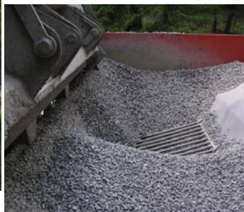
Figure 20. Receiving hopper of the chip spreader as the truck dumps.
