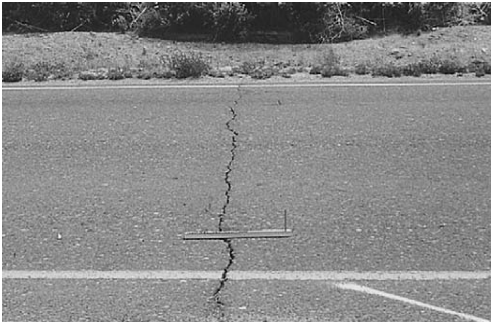
FIGURE 6 Thermal cracking.
