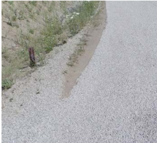
Figure 21. Note that extra chips are swept to the roadside.
