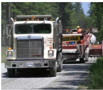
Figure 19. The aggregate truck putting down 20 to 30 lb/SY application rate of 1/2" to No. 4 chips.
