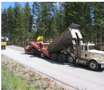
Figure 26. Applying the choke stone.
