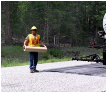
Figure 42. When ready to restart construction, paper is needed.
