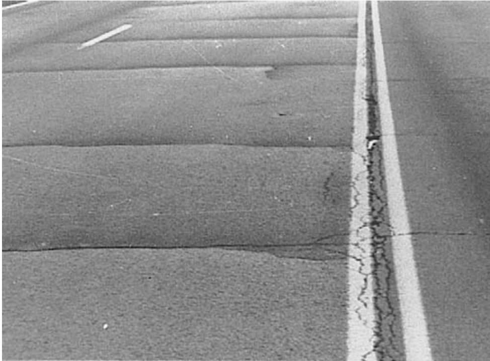
FIGURE 11 Reflection cracking.
