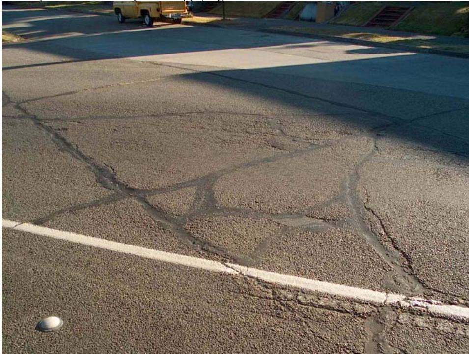
Figure 31: Crack sealing in western Oregon to repair transverse cracks.
