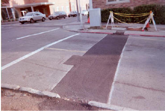
Figure 27: Full-depth patch.
