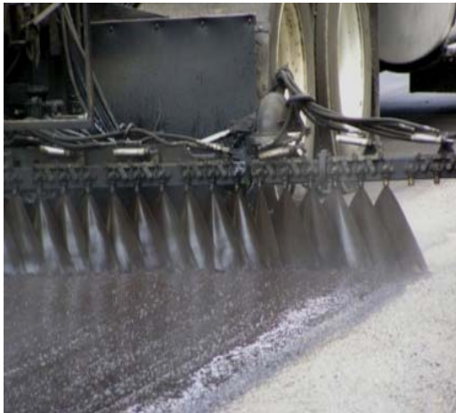
Figure 10. Close-up of asphalt emulsion being sprayed onto a prepared surface. The spray bar allows for consistent coverage of one lane-width at a time.
