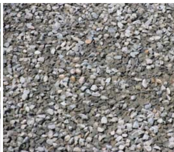
Figure 27. Close up of BST after choke stone application. Note tighter surface almost completely covering underlying asphalt.
