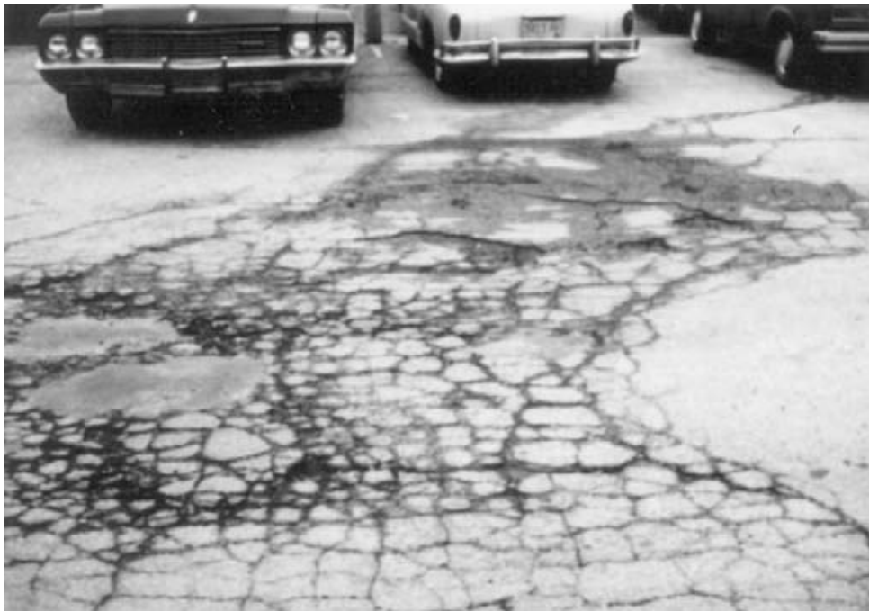
FIGURE 14 Reflection cracking.
